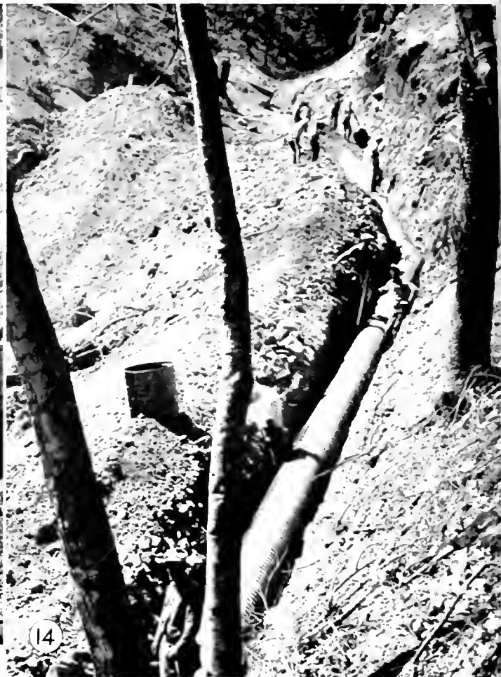
Figure 13a. Bottom Location—reinforced concrete arch on curved alignment and uniform gradient in bottom of ravine. Figure 13b. Bottom Location—reinforced concrete arch on straight alignment and broken gradient. Figure 14. Modified Bottom Location—corrugated metal pipe, with entrance in bottom of ravine and alignment following grade tour in sidehill trench, to an outlet well above and to one side of natural channel.
